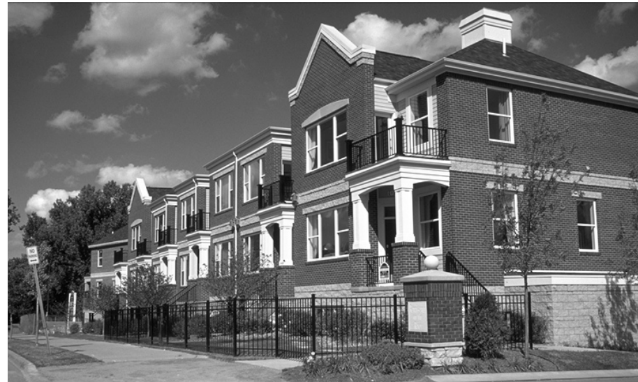
These townhouses were developed with such distinct design elements as front porches and horizontal expression lines in a material that contrasts the brick facade and matches the building's stone base.
