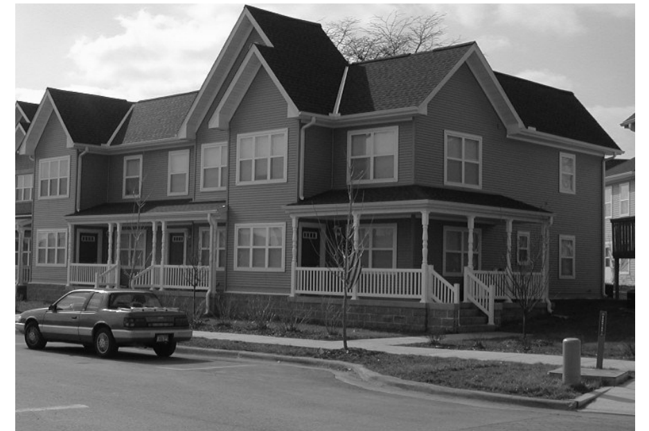
Porches wrapping into corner side yards and transparency, coupled with different gabled roofs, make this building interesting, whether one is passing along the front or side facades.
