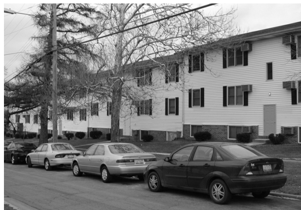
Existing apartment buildings on Broadway Avenue.
