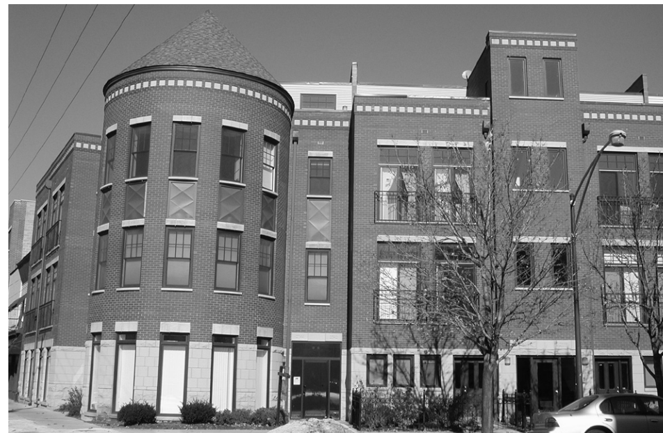
Vertically oriented windows with metal accents and varied roof types provide interest to the brick and stone facade of this apartment building.
