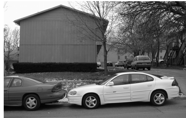
Existing apartment building on Broadway Avenue.
